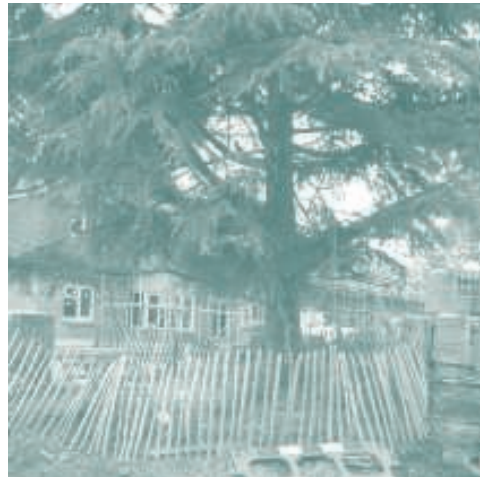
Inadequate protective fencing leads to tree roots being damaged
